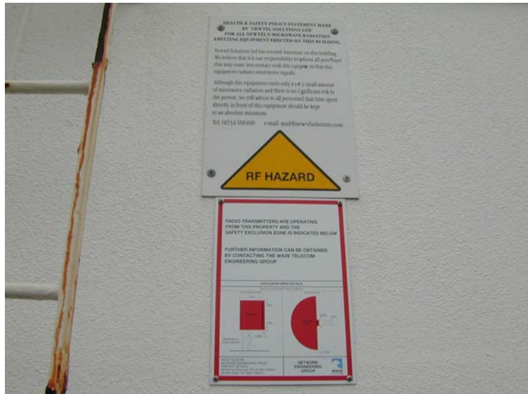
Figure 2 Photograph of poster by the Beau Sejour antennas (Newtel and Wave signs)
